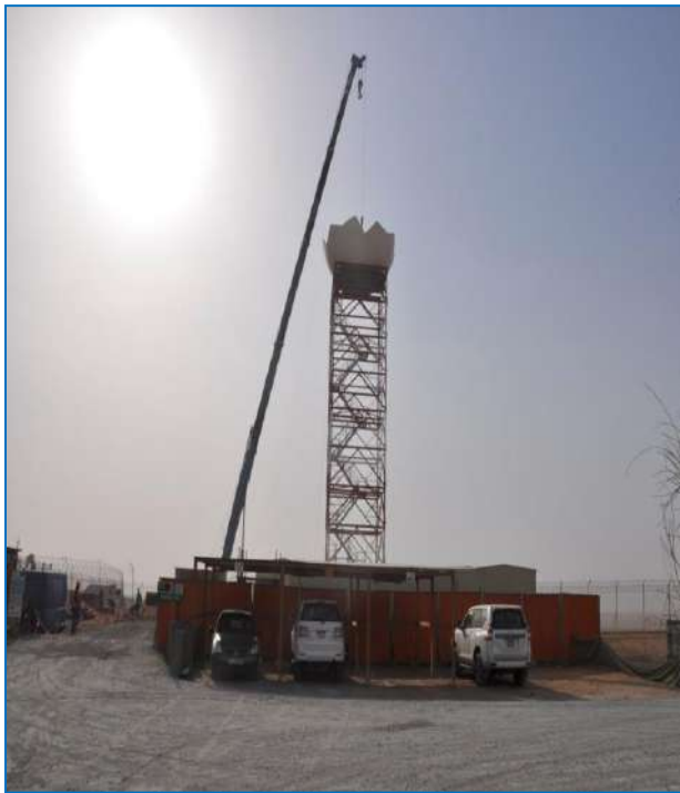
Installation of Radar Tower and Radom
