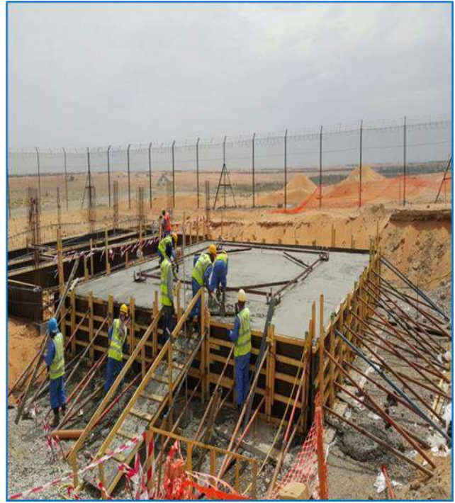
MSSR Radar Tower Foundation works
