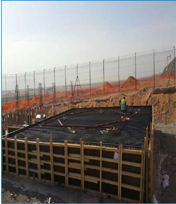
MSSR Radar Tower Foundation works
