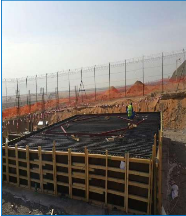
MSSR Radar Tower Foundation works
