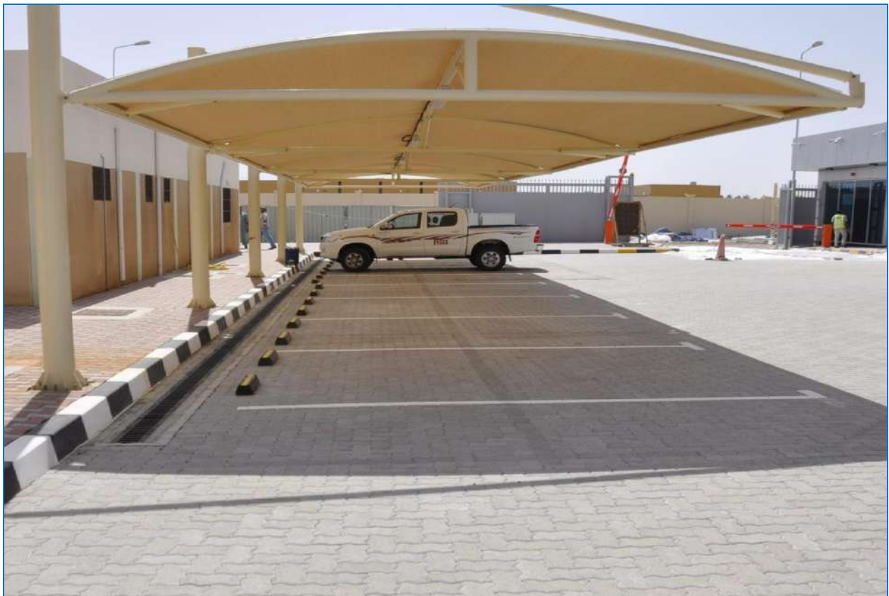
Car shade and Interlock works at Gate House
