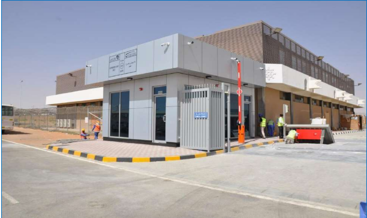
Gate House Building
