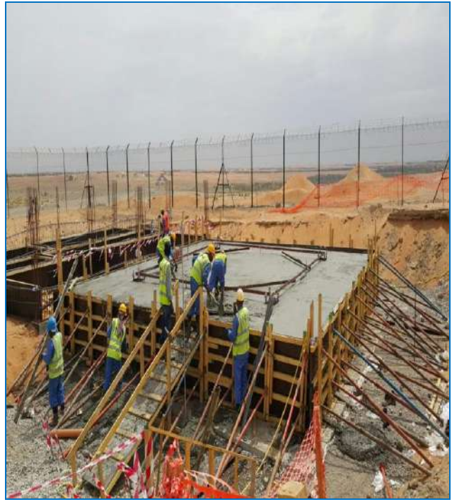
MSSR Radar Tower Foundation works
